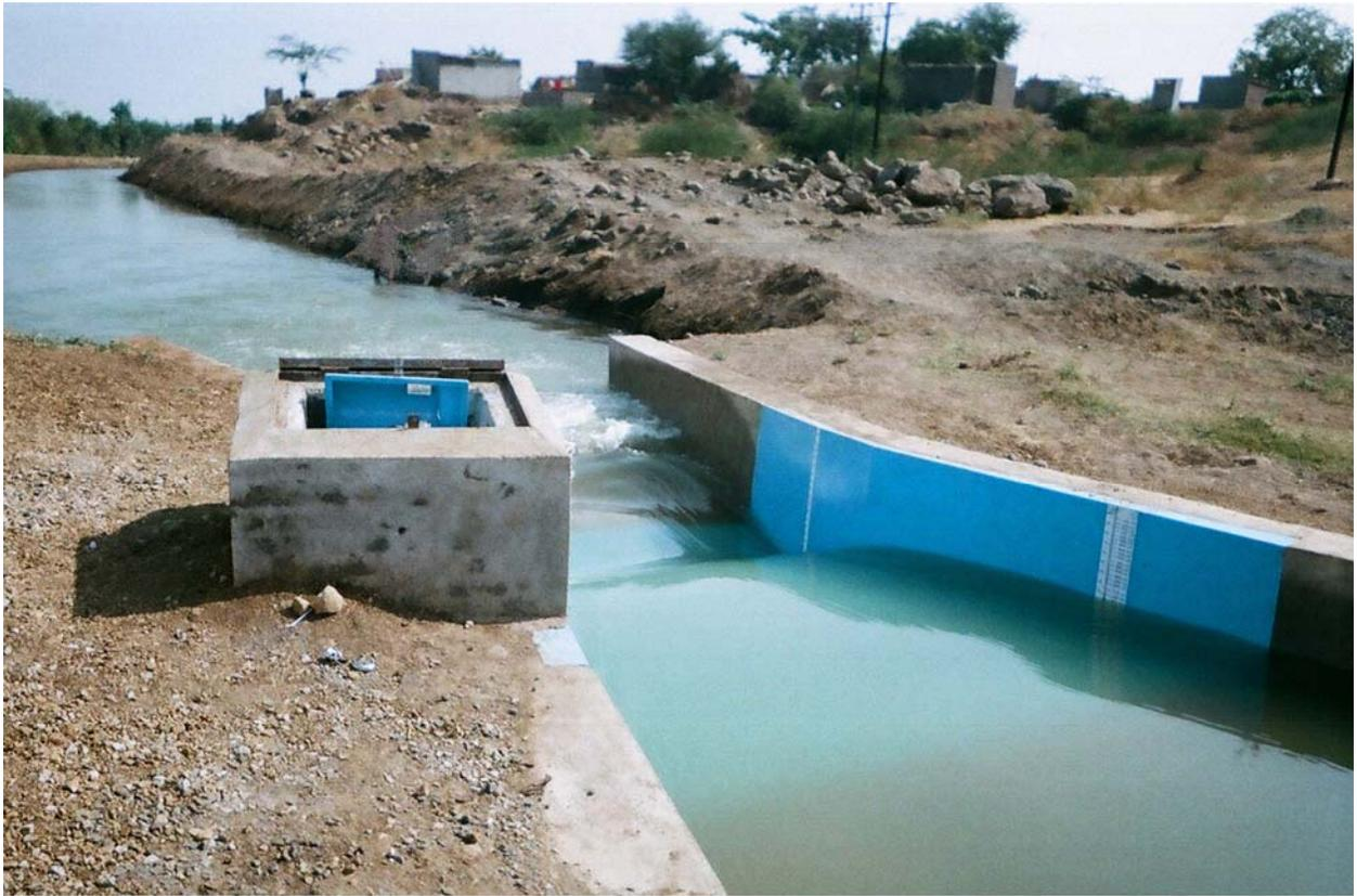
Parshall Flume Of 150 Cusecs Capacity With Digital Water Stage Recorder @ ch 0/400 of Mangi Right Bank Canal Of Mangi Medium Project Tal.Karmala Dist.Solapur.
