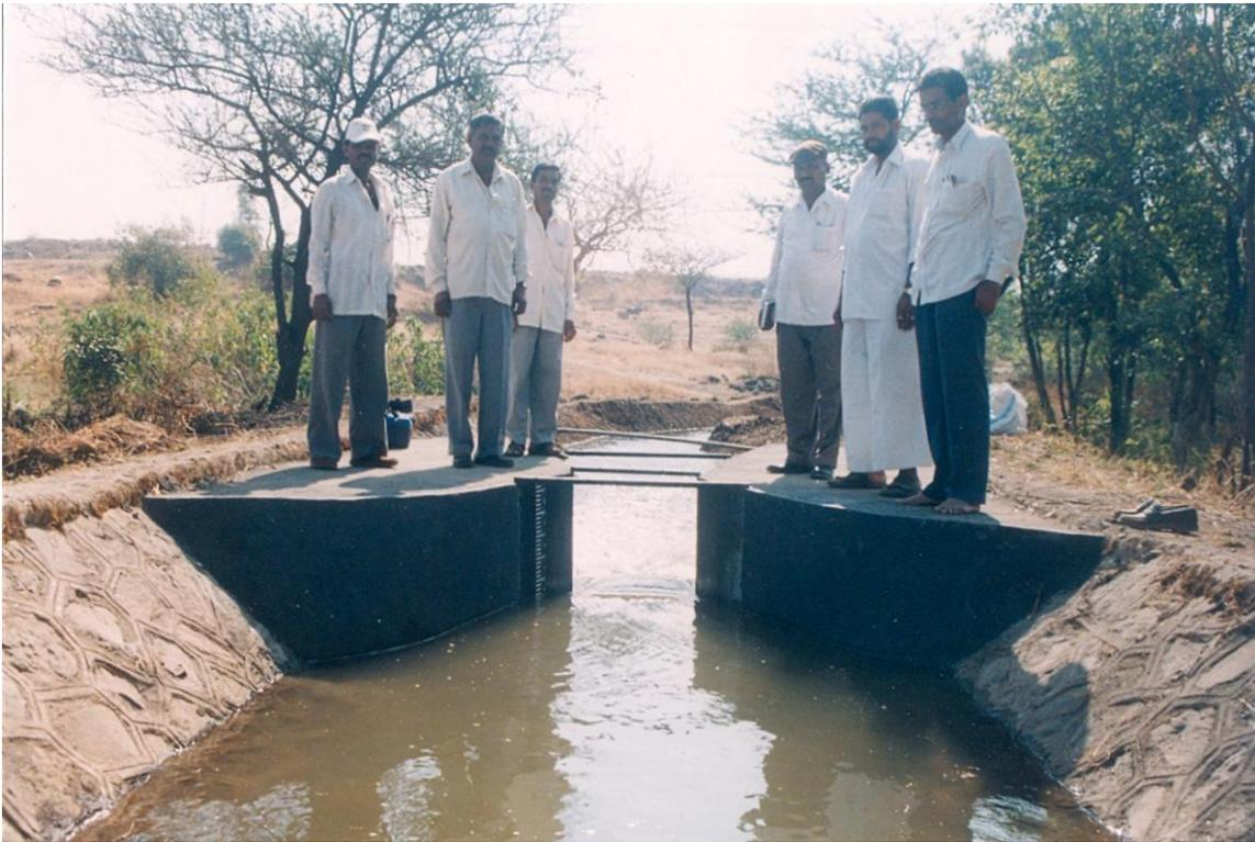
Cut Throat Flume of Left Bank Canal of Diwale MI Project
